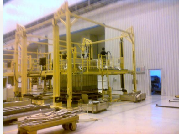
Coil Assembly Platform
